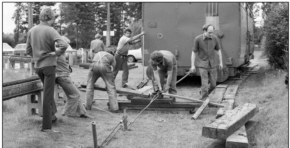
*Success! The van is on its way inch by inch towards its destination. The sleepers forming the 'plateway' and rollers are clearly visible behind Dick on the right.*
